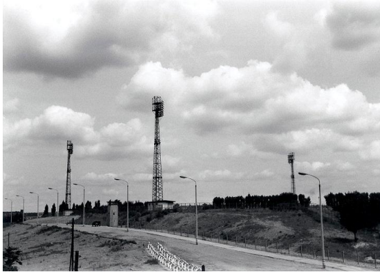
Border strip 1968 in the later Mauerpark
